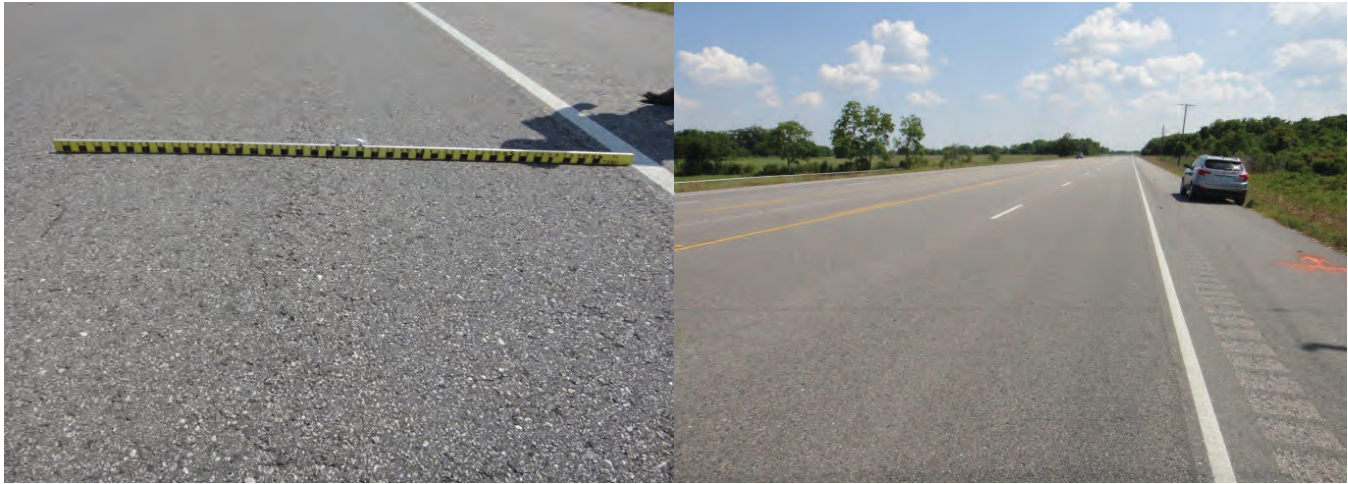
Figure 8-3. Good Condition of the RAP/RAS Test Section on SH 146, Houston.
